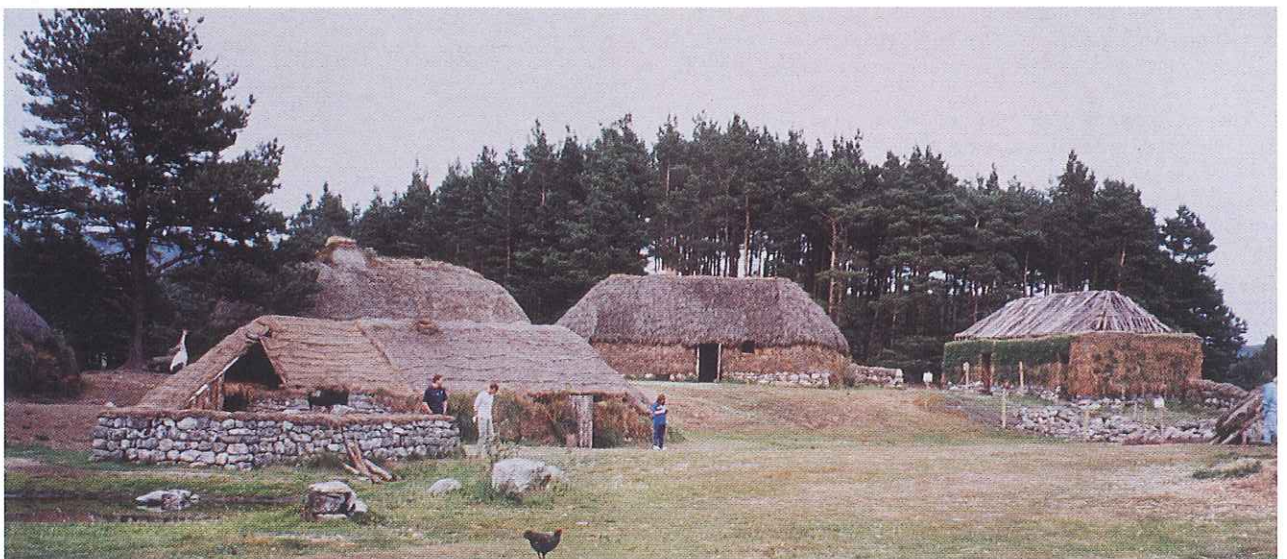
The reconstruction of post-medieval buildings on the Highland Folk Park, Newtonmore, has an important role for education, recreation and tourism, and in our understanding of how these buildings were built and used.
