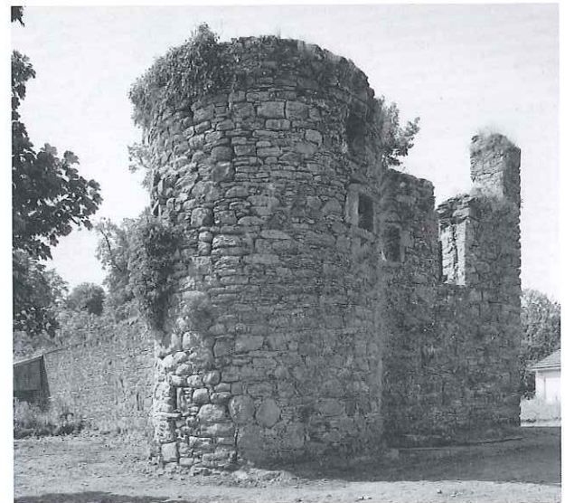
The ruins of Gartartan Castle stand in the grounds of Gartmore House, on the edge of the Forth valley. The castle walls were extensively robbed to provide stone for a walled garden in the eighteenth century (NMRS C7253).
